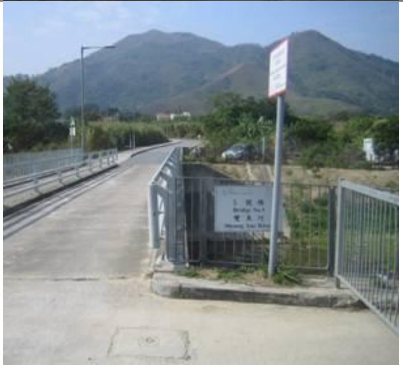
11. Bridge No.5 Sheung Yue River 雙魚河 5 号橋
